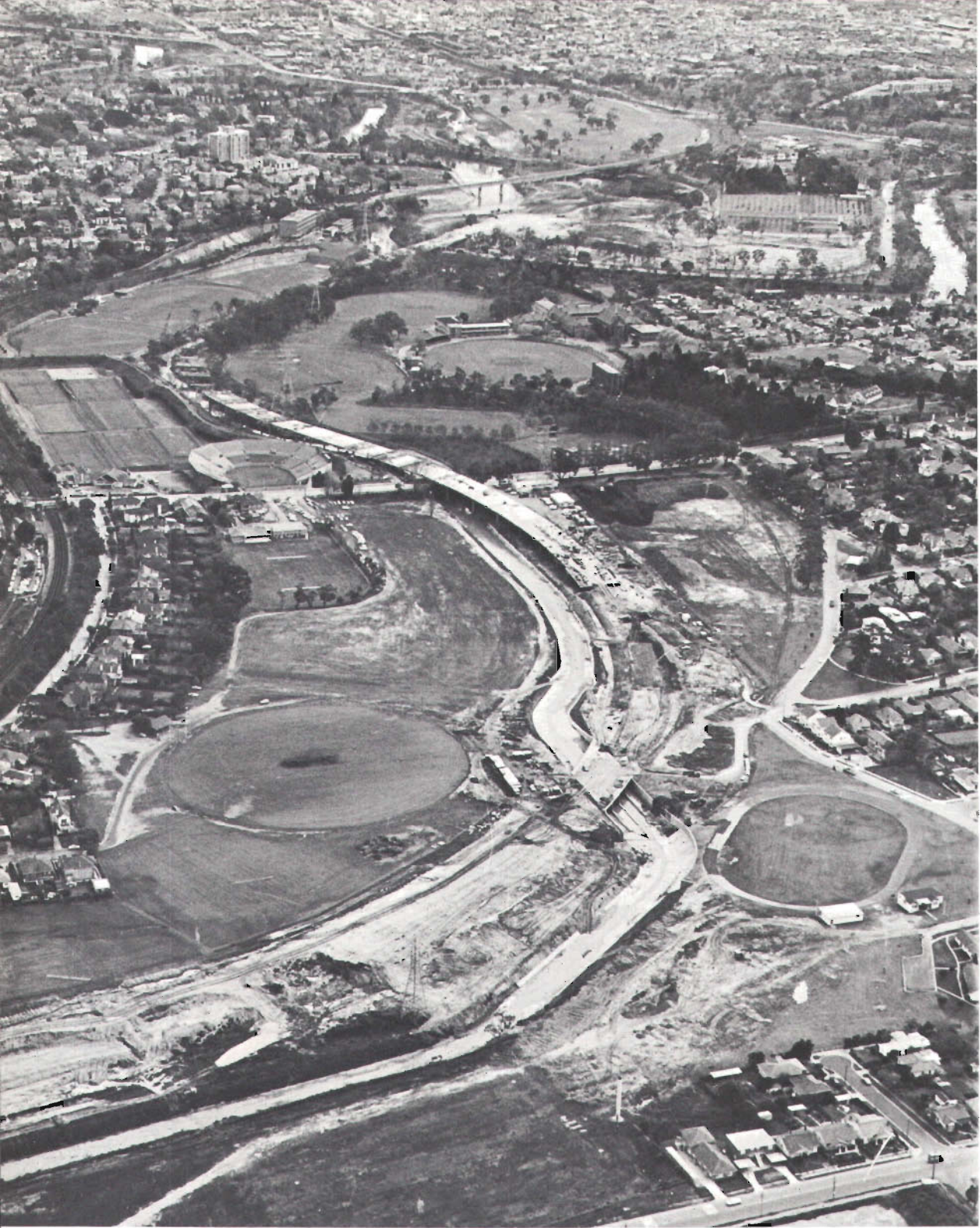
The second stage of Melbourne's South Eastern Freeway shown under construction in October 1969.
