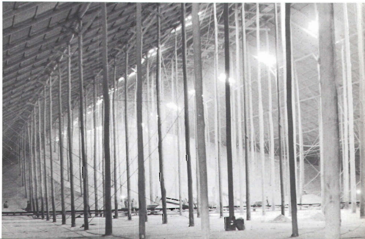
The interior of the bulk wheat storage at Dunolly, in the Wimmera, which has a capacity of 10.5 million bushels. The roof is supported by 1,320 imported timber poles.
